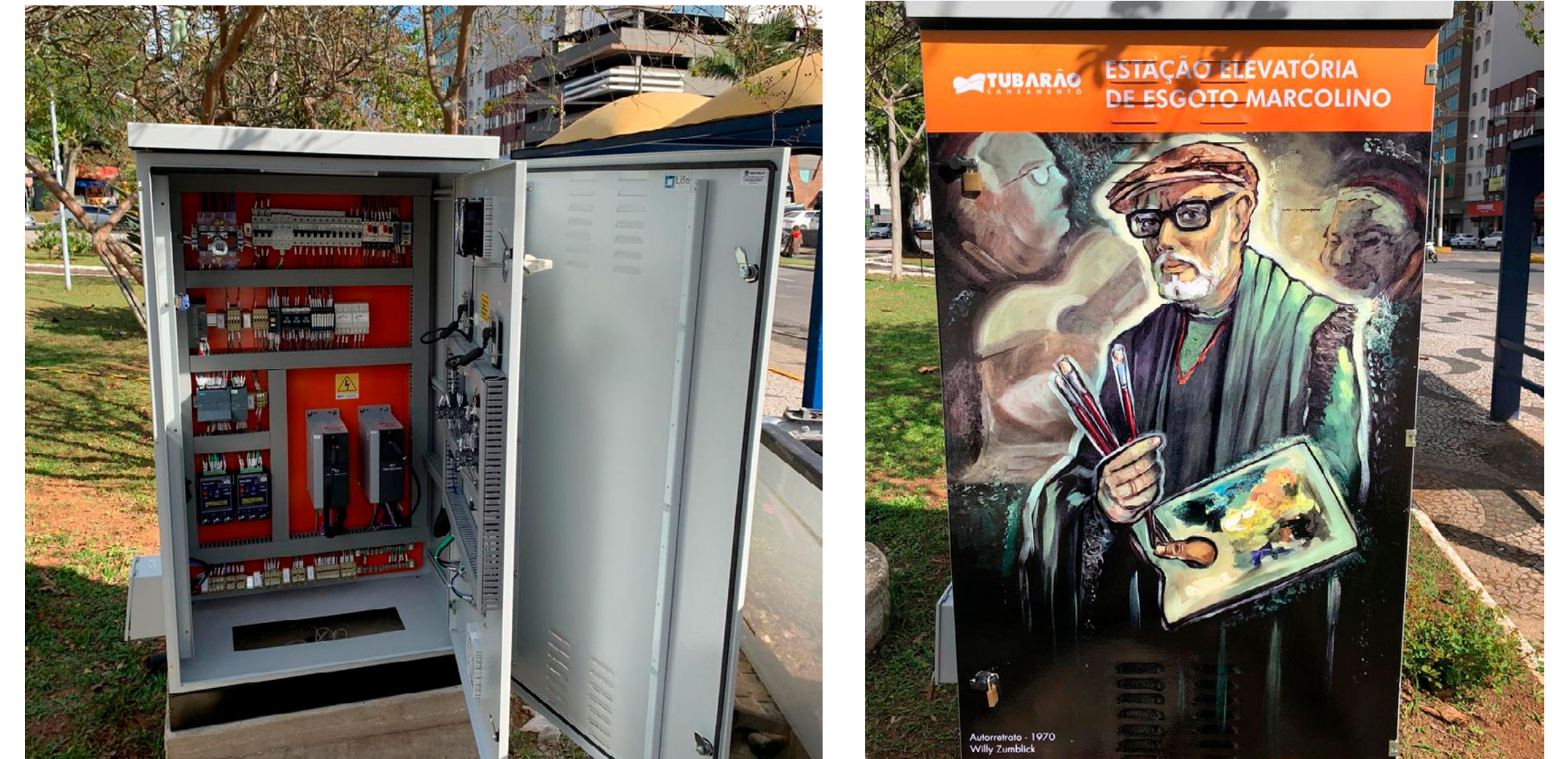
Details of the inner part (on the left) and of the door (on the right) of the SPS control panel
